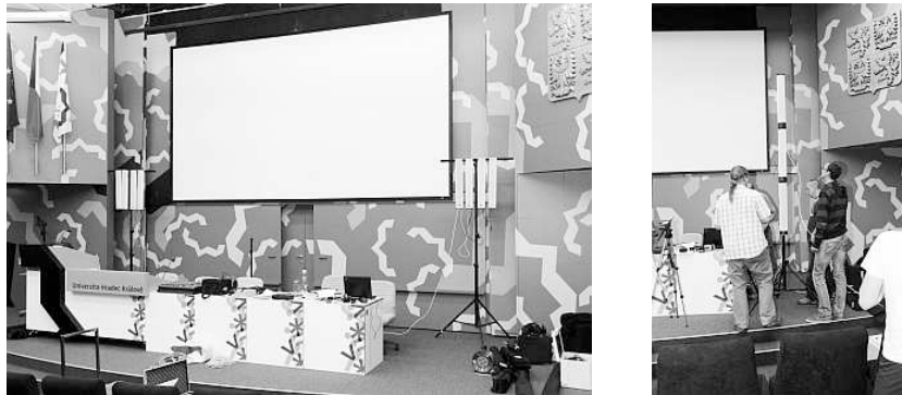
Fig.7 Wall speakers and two-meters column speaker in assembly hall of University of Hradec Kralove
