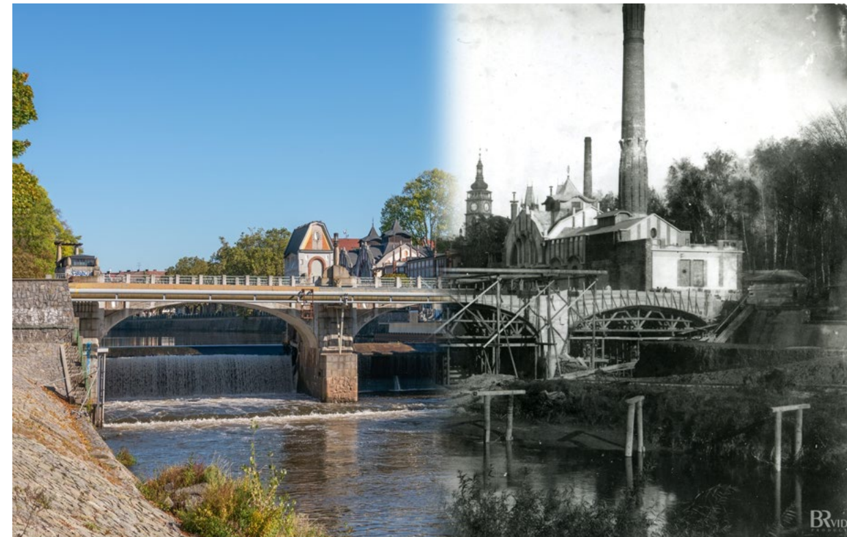
HUČÁK: AN ART NOUVEAU STYLE POWER STATION (CULTURAL MONUMENT) AND A BRIDGE OVER THE ELBE RIVER NEAR THE JIRÁSKOVY SADY PARK, TURN OF THE 20 TH CENTURY
