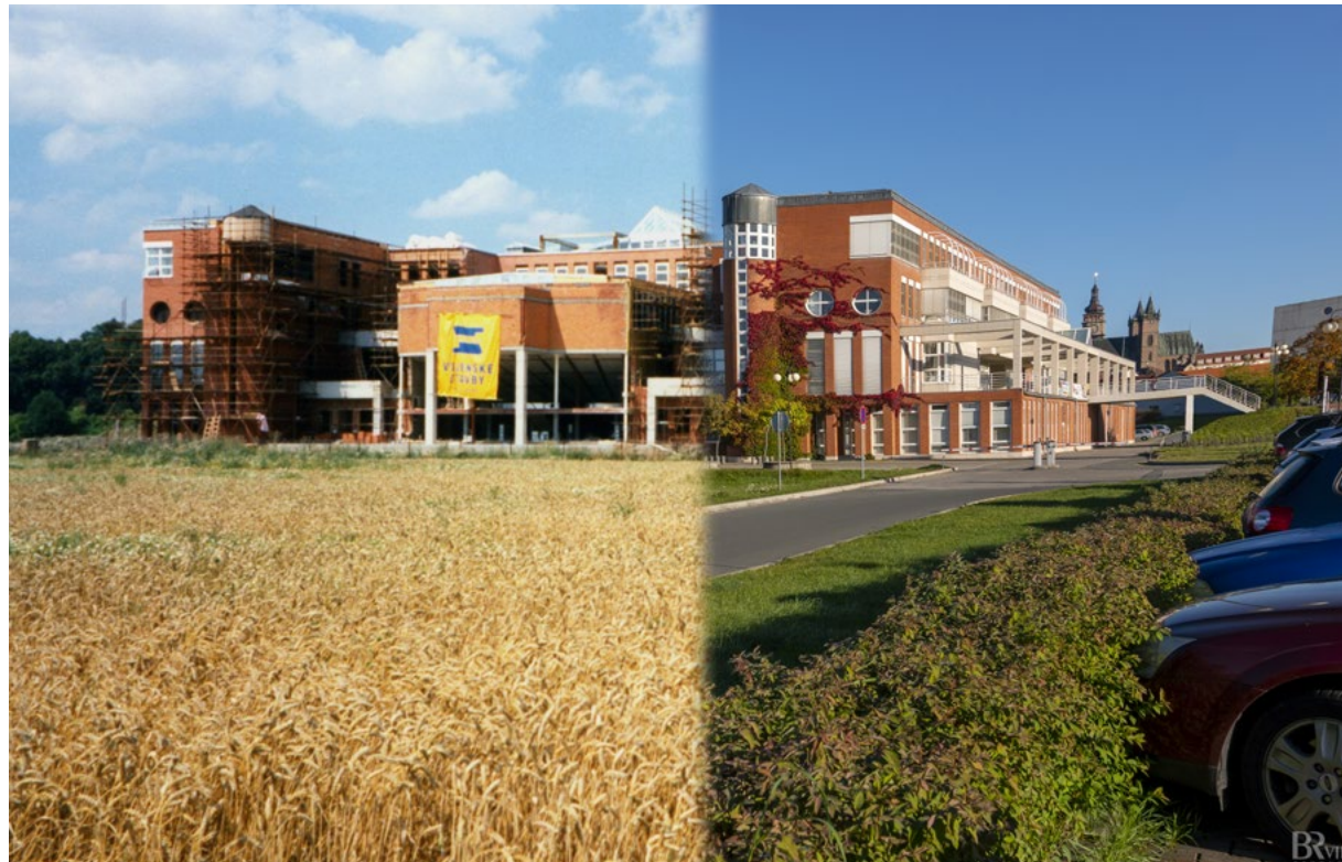
UHK BUILDING OF COMMON EDUCATION UNDER CONSTRUCTION, 1996
